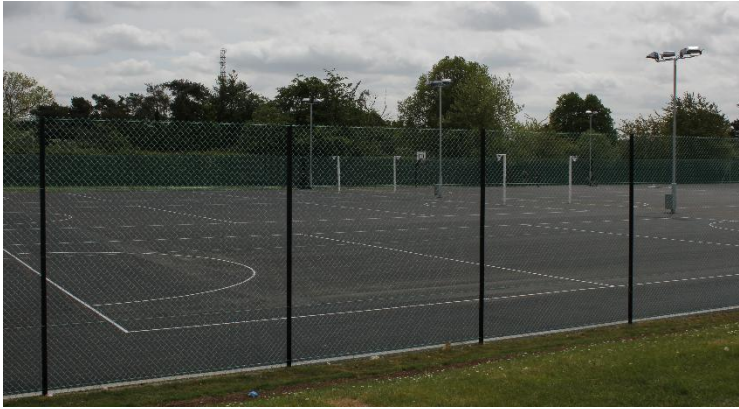
Figure 2: redevelopment of netball courts at Stanborough School
